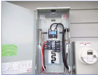
A. Item 2(Picture) main panel - interior
