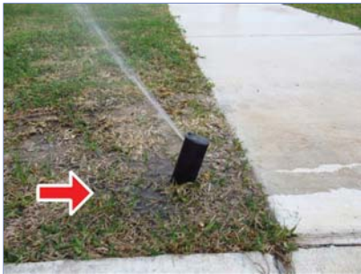
A. Item 3(Picture) tilted head / possible under ground leak
