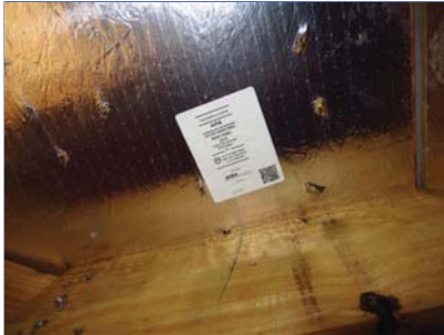
D. Item 1(Picture) radiant barrier
