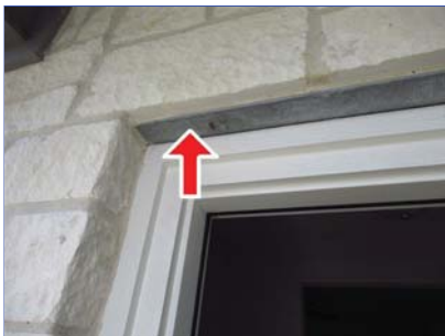
E. Item 4(Picture) exposed lintels
