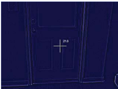
D. Item 1(Picture) rear door - well sealed
