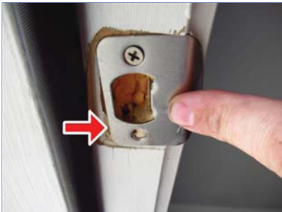
G. Item 2(Picture) striker missing screw
